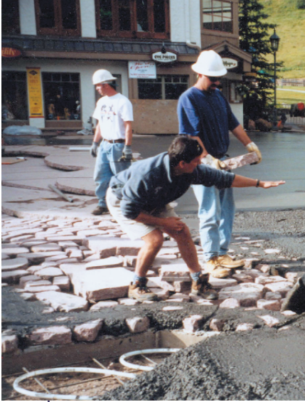
Seibert Circle Construction
