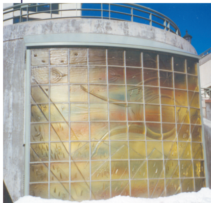
Exuberance Village Parking Structure
