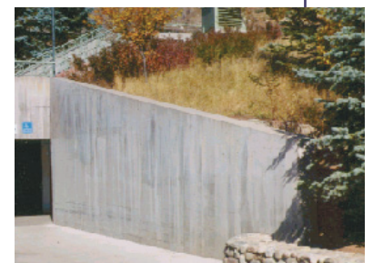
Vail parking structure wall
