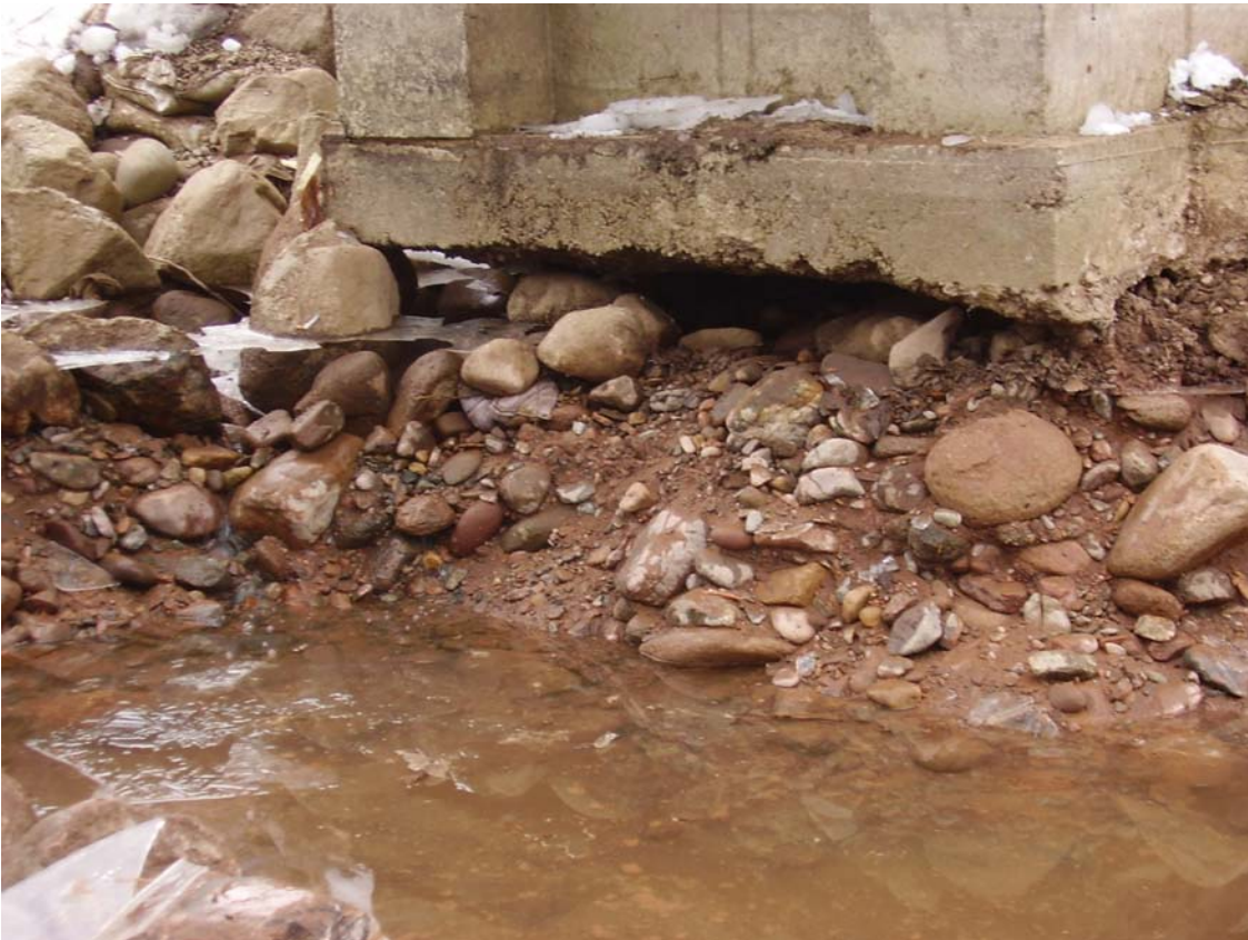
South abutment Christopher Sewell Bridge inspected December 6, 2010, Vail, CO
