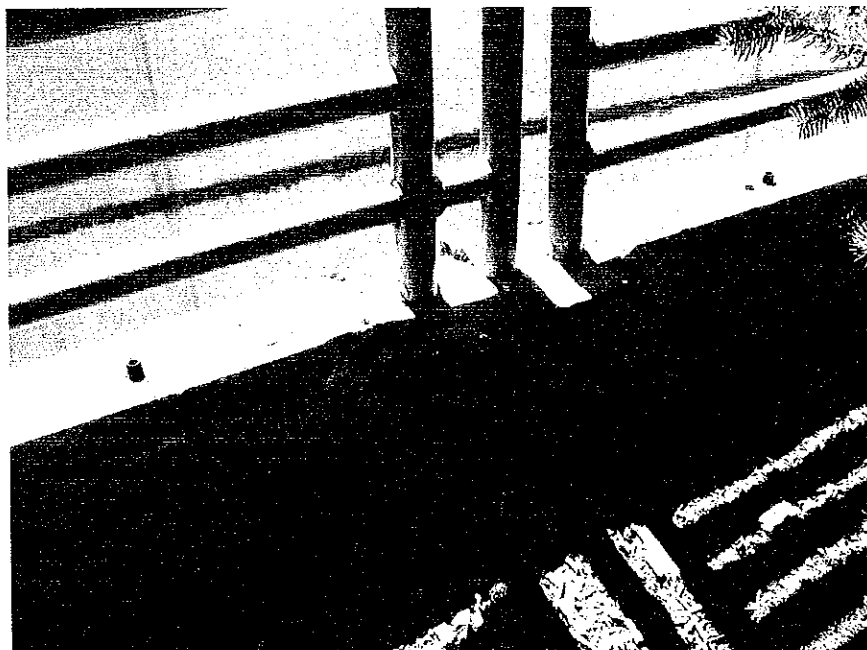
Photo 14. Connection of railing post to concrete wall is deteriorated. This is a typical condition along C from 20 to 30. The connection should be repaired.
