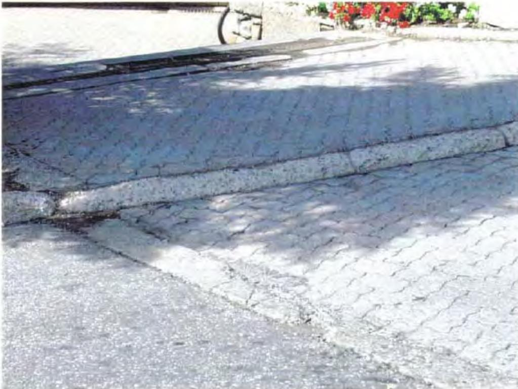
*Figure 3-21a- Disrepair of concrete pavement and paverstones*
