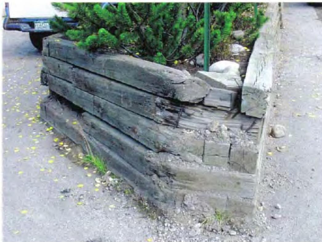
*Figure 3-19a- Typical disrepair of retaining walls and planters*
