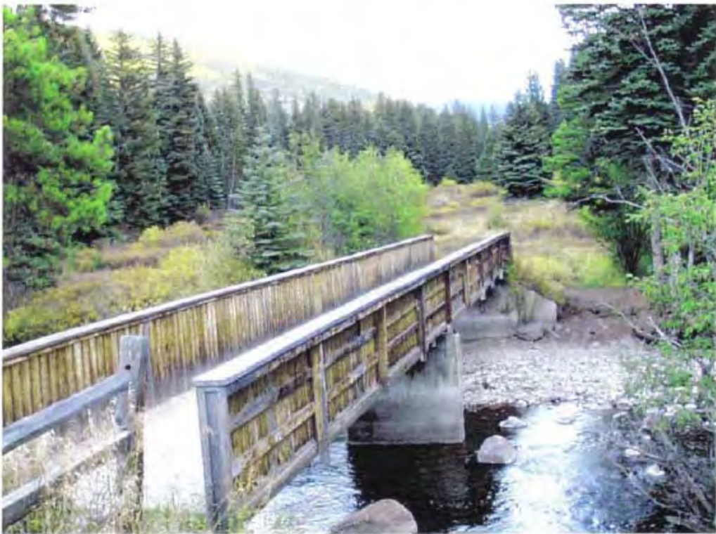
Figure 3-3b- Footbridge across Gore creek to wetland area
