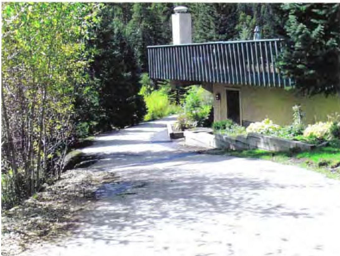
Figure 3-13- Pedestrian path and pool deck conflict area behind Antlers condominiums
