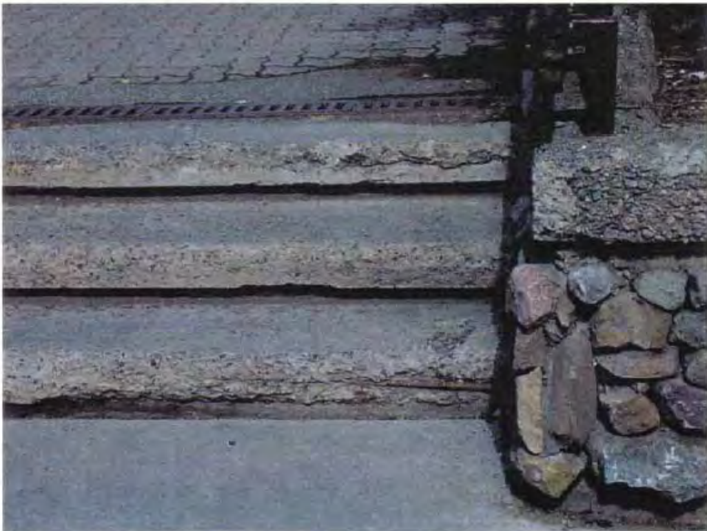
Figure 3-21b- Typical condition of concrete steps and stone cheekwalls
