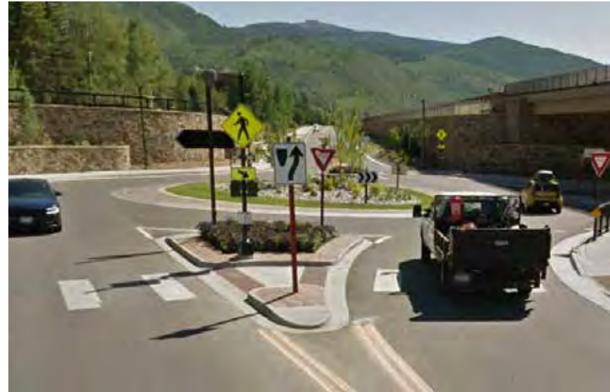
Roundabout at the Simba Run underpass
