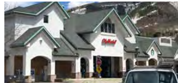
Vail Commons includes a 50,000 square foot City Market with one of two pharmacies in Vail
