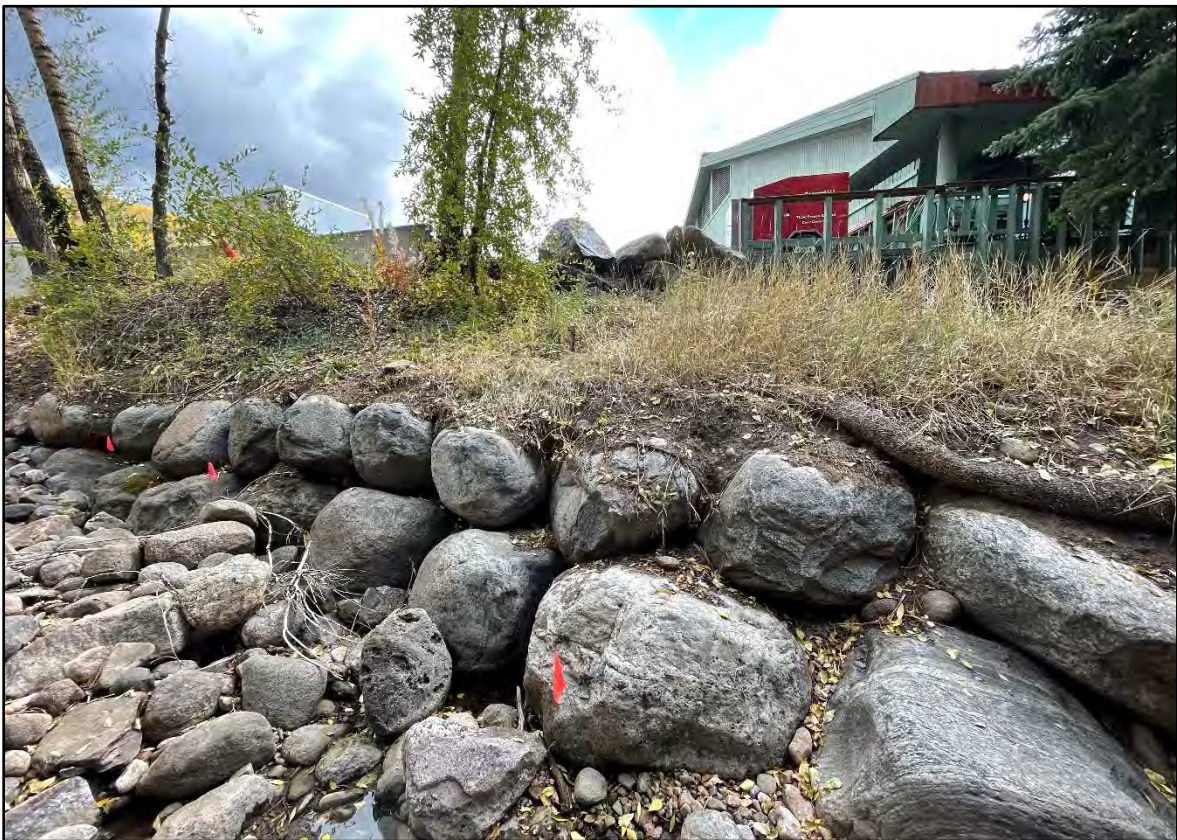
Photo 4. Boulder bank treatments along the upper part of the reach with a low cover of desirable riparian plants. (9/28/21).
