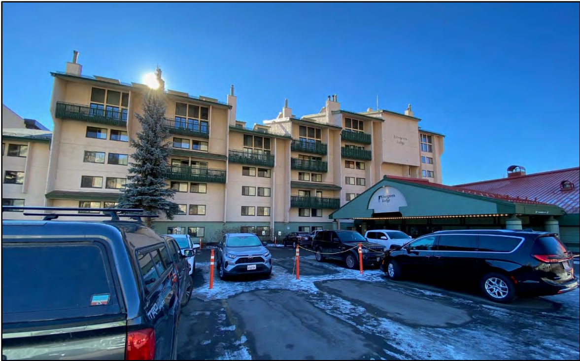
Photo 1. View of the exterior of the Evergreen Lodge and paved parking area north of the building. (12/7/21).
