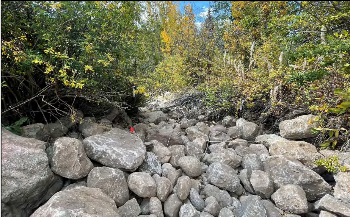
Photo 5. Recently placed cobble and riparian vegetation along the upper reach. (9/28/21).
