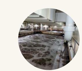
**AERATION** Air is added to a mixture of wastewater and bacteria, which digest harmful organic waste.
