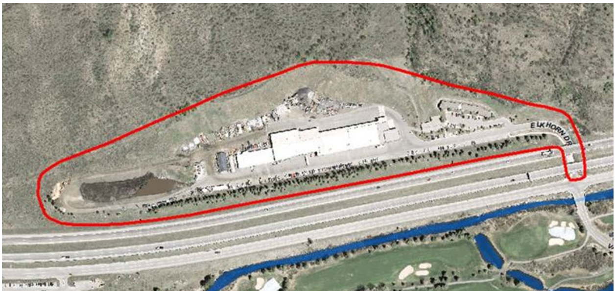
(Public Works site, approximately 17.3 acres)
