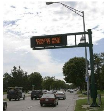
Photo 7 – Overhead DMS example
