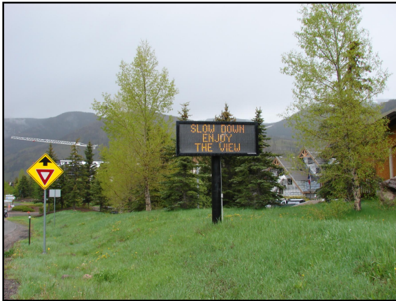
Photo 1 - Existing I-70 Off ramp DMS
