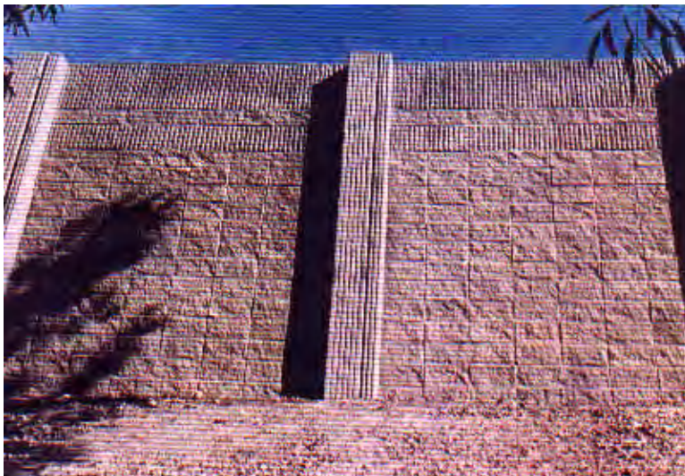
Masonry Form Liner Wall
