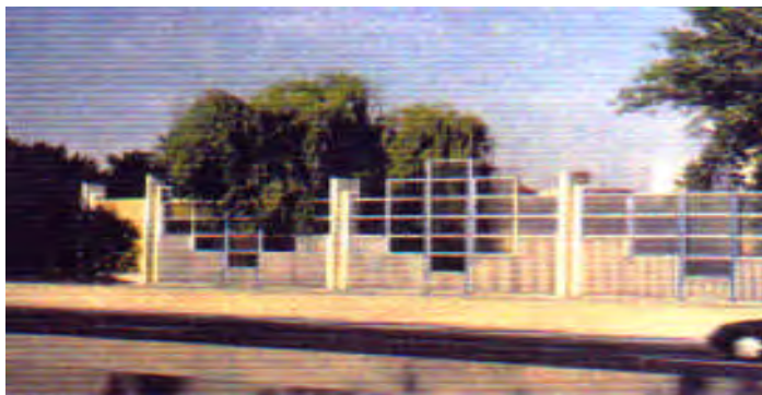
Glass Noise Wall, France
