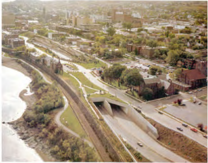
Cut-and-cover tunnel; Duluth, Minnesota
