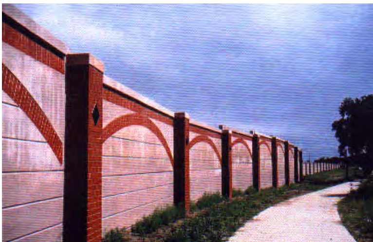
Masonry Form Liner Wall I-25, Colorado Springs, (neighborhood side)
