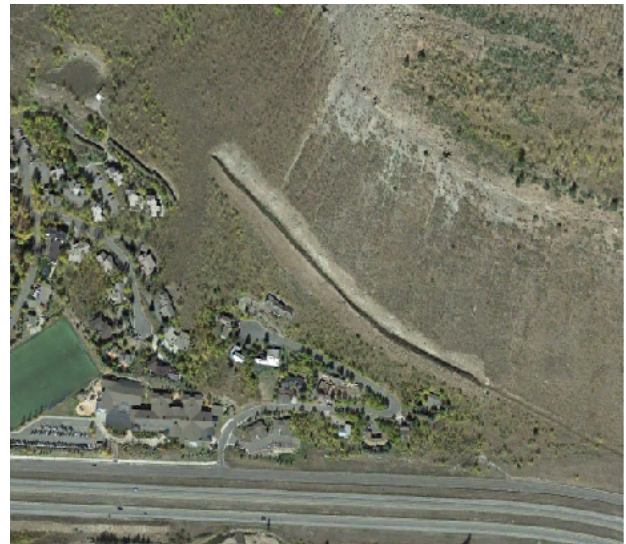
Booth Falls rockfall mitigation berm
