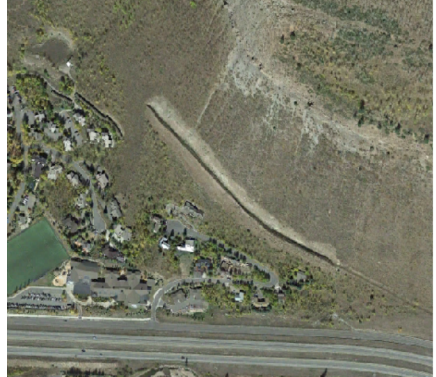
Booth Falls rockfall mitigation berm
