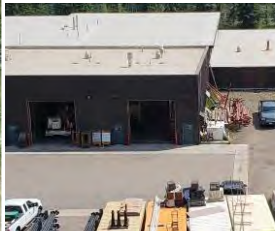
View from 2 nd utility transformer feeding the Maintenance building.
