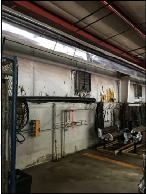
Photo 2: Tension Only Steel Cross Brace
