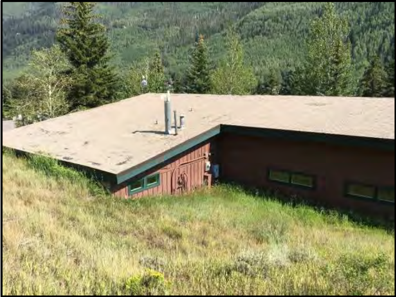
Photo 1: North Side of Administration Building Looking South
