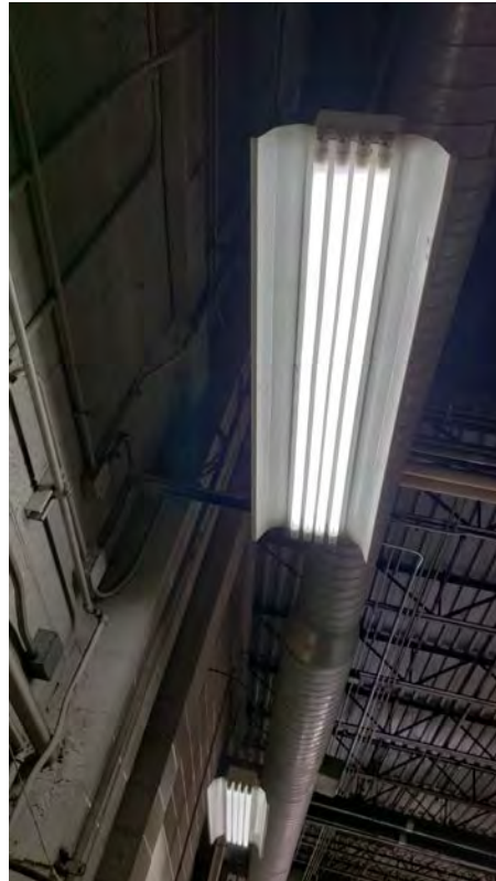
Maintenance Building industrial Fluorescent fixture retrofit with LEDs
