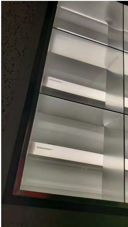
Maintenance and Admin Building typical Fluorescent fixture retrofit with LEDs
