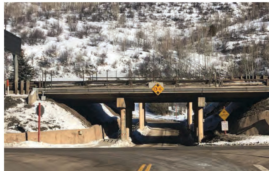
UNDERPASS APPROACH LOOKING NORTH
