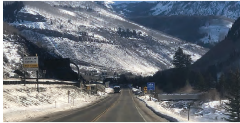
FRONTAGE ROAD LOOKING EAST GORE CREEK ON THE RIGHT
